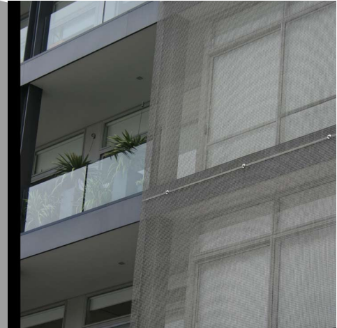
* Typical Architectural Installation
